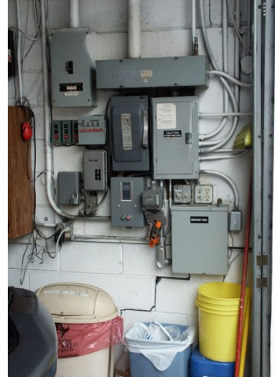
Figure 2 (left) shows cracking in the top right corner above door frame, loose barrier above door and smoke and fire penetrations in walls and ceilings. Figure 3 (right) shows severe cracking below and behind electrical panels. Storage of flammable materials around electrical panels.
