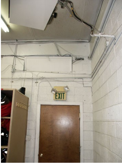
Figure 2 (left) shows cracking in the top right corner above door frame, loose barrier above door and smoke and fire penetrations in walls and ceilings. Figure 3 (right) shows severe cracking below and behind electrical panels. Storage of flammable materials around electrical panels.
